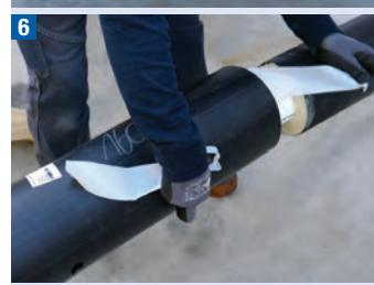
The sealant bands are already pre-applied inside the heat-shrinking casing pipe. Remove the protective paper inside. Place the heat-shrinking casing pipe by paying attention that its ends overlap on the sealants bands.
