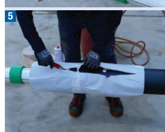
Remove the packaging of the heat-shrinking casing pipe by using a cutter. Do not damage the pipe casing.
