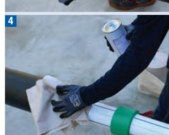
Clean the ends, which were previously ground with the cleaning liquid (item 50330), and then perform a preheating operation by using the torch up to about 40° in the area to be coated.
