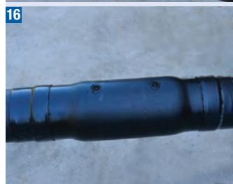
After performing the cleaning operation with the cleaning liquid (item 50330), remove the packaging film from the shrinkable band, and then place it on the welding of the casing pipe by paying attention that the middle line of the band correspond to the welding line.
