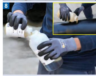
Mix the bicomponent products by pouring the polyol content into the isocyanate container: after that, shake quickly for a few seconds, and then pour the content into one of the two holes.
