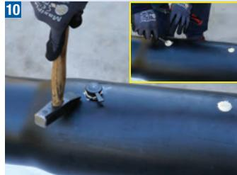
With a light hammer blow, pop the drilled curing caps. The hardened foam will look like the picture in the yellow box. With a rasp, slightly scrape the material to remove foam residues; after that, wipe with a cloth soaked in the cleaning liquid (item 50330) to finish the cleaning operation.
