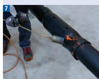
Heat the heat-shrinkable band evenly; the band will start acting as glue. At the end of the operation there will be a slight leakage of sealing material at the sides of the heat-shrinkable band. Repeat the operation for both heat-shrinkable bands.
