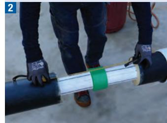
Measure the length of the casing pipe and subtract the length of the non-insulated pipe from the detected measure. Divide the result by two: the obtained measure must be measured from the end of the pre-insulated pipe and marked with a white marker so that the position of heat-shrinking casing pipe ends will be clear.
