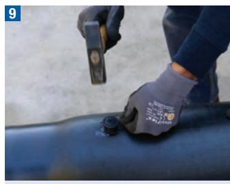
Place the two supplied curing caps by paying attention that the vent opening is not pushed inside the hole. After that, wait for about 5-10 minutes, in relation to the outside temperature, so that the introduced mixture becomes foam.
