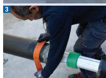
By using emery cloth (sandpaper), abrade the pre-insulated pipe by about 0,1 ÷ 0,25 mm by rubbing its end: start from the drawn line towards the inside to remove impurities and the oxidized layer of the insulator. Repeat the operation on both sides.
